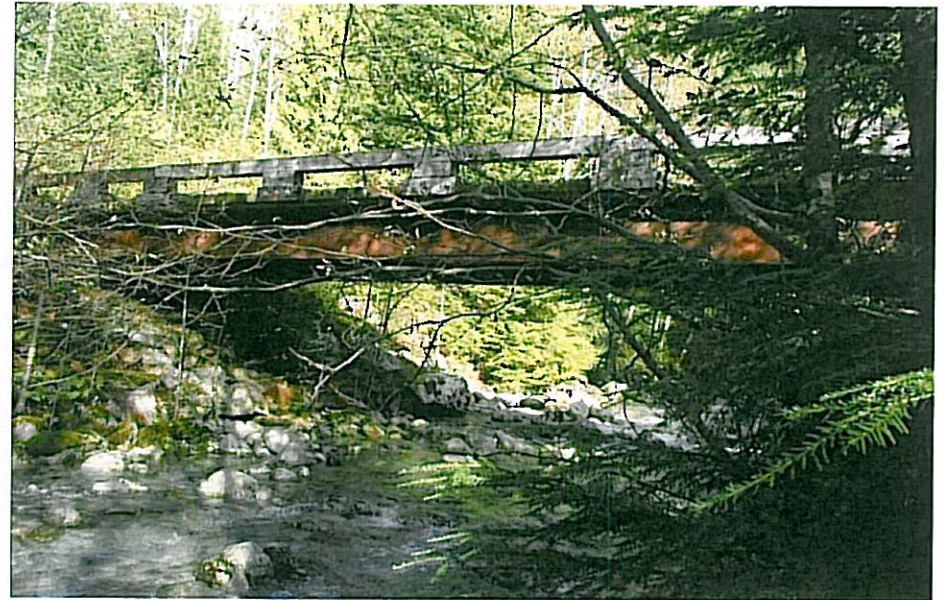
CK-2345 From Downstream
