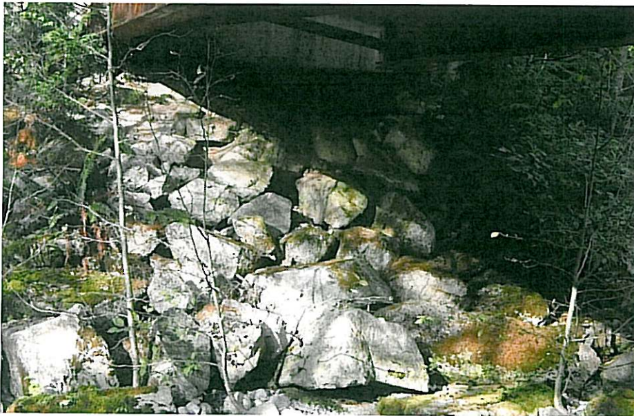
CK-2345 Right Abutment
